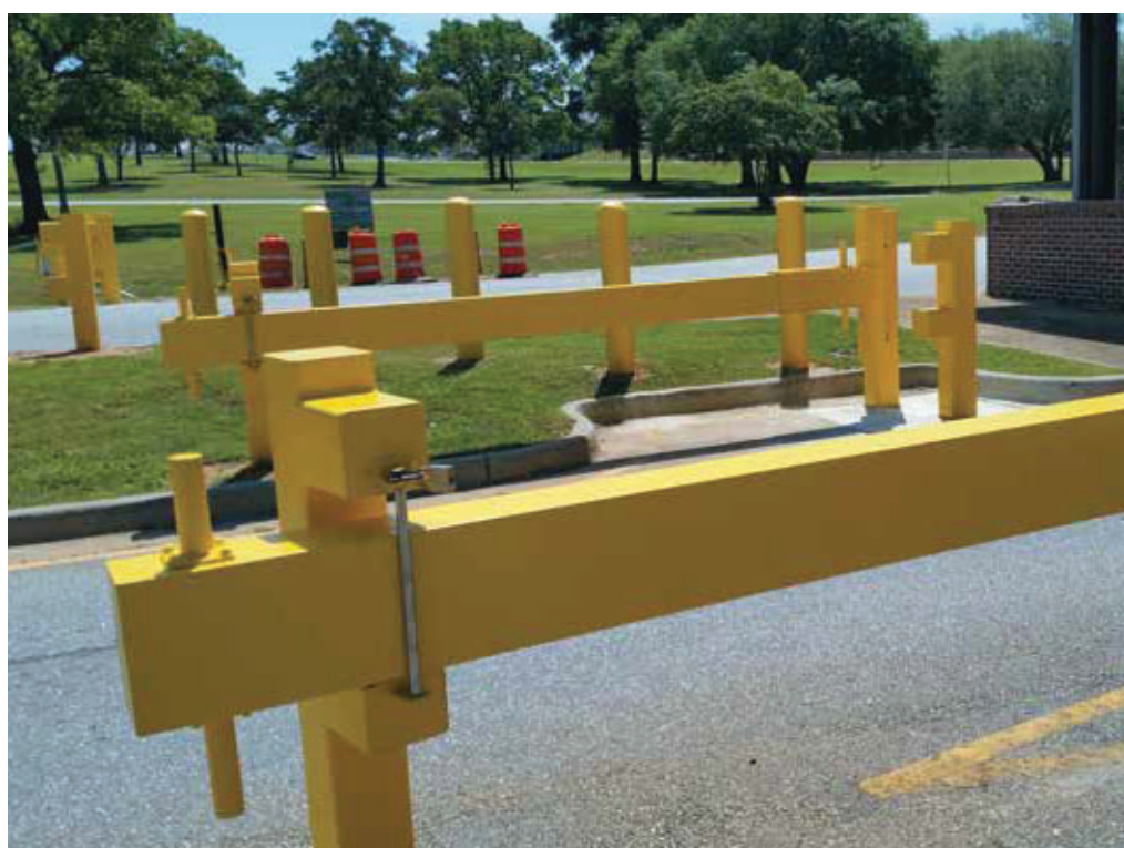
Crash-rated manual swing arms, seen here in the open position, are the most economical form of crash-rated active barrier.
