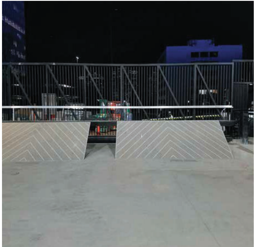
A wedge barrier viewed from the secure side. IMAGE COURTESY OF AMICO SECURITY
